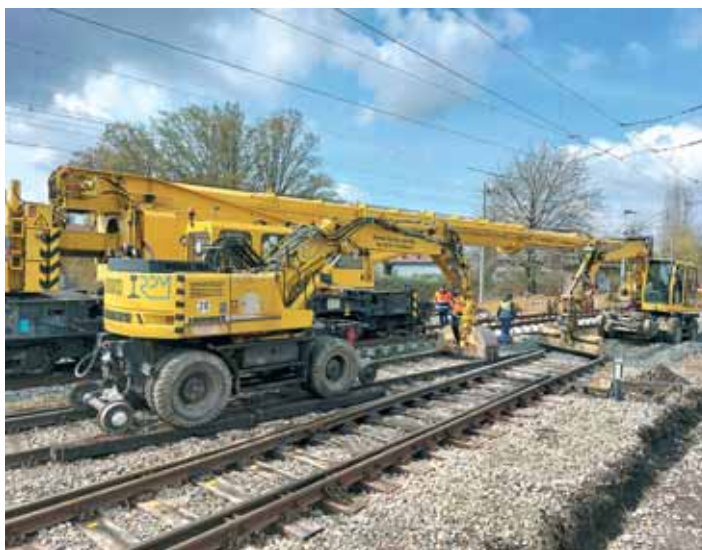
Radovi u kolodvoru Podsused
