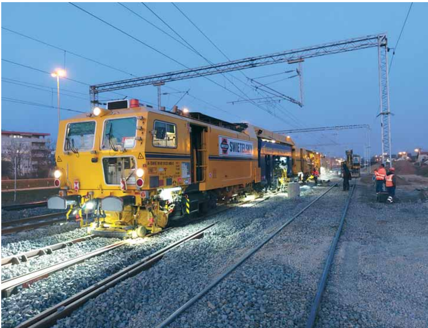
Radovi u kolodvoru Podsused
