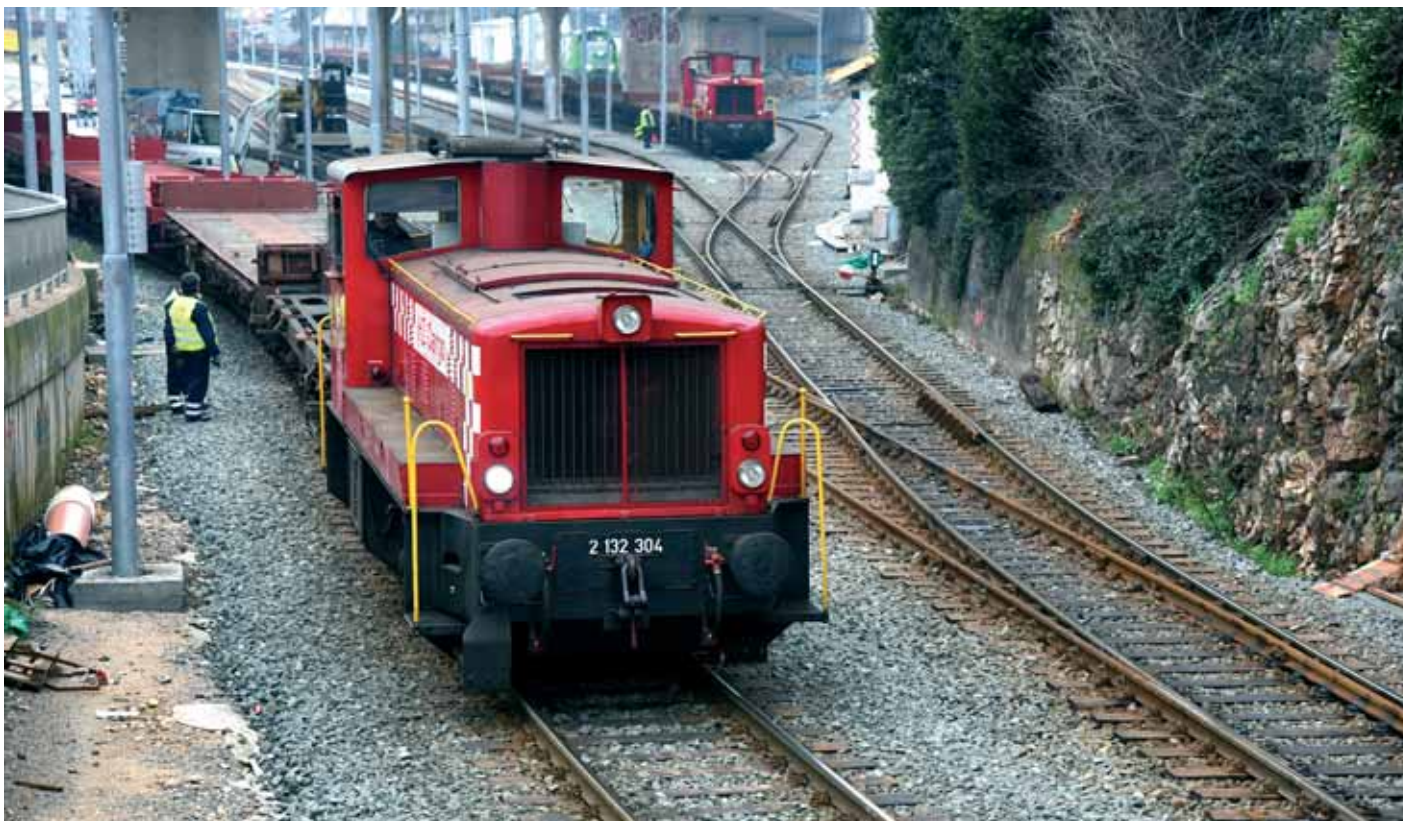
Manevarski rad ispred tunela
