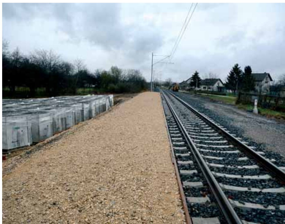
Remont pruge Greda – Sunja
